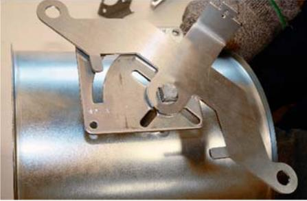
1. Place the swivel arm on the axle in the desired position depending on the position of the throttle valve in the installation,
